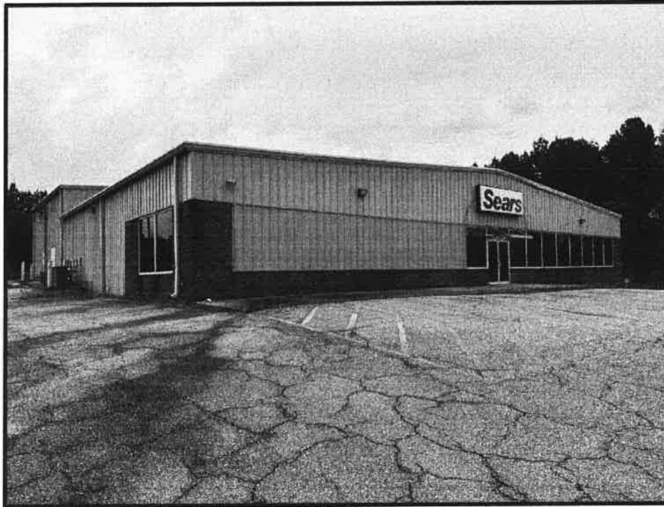
Front view and southern elevations
