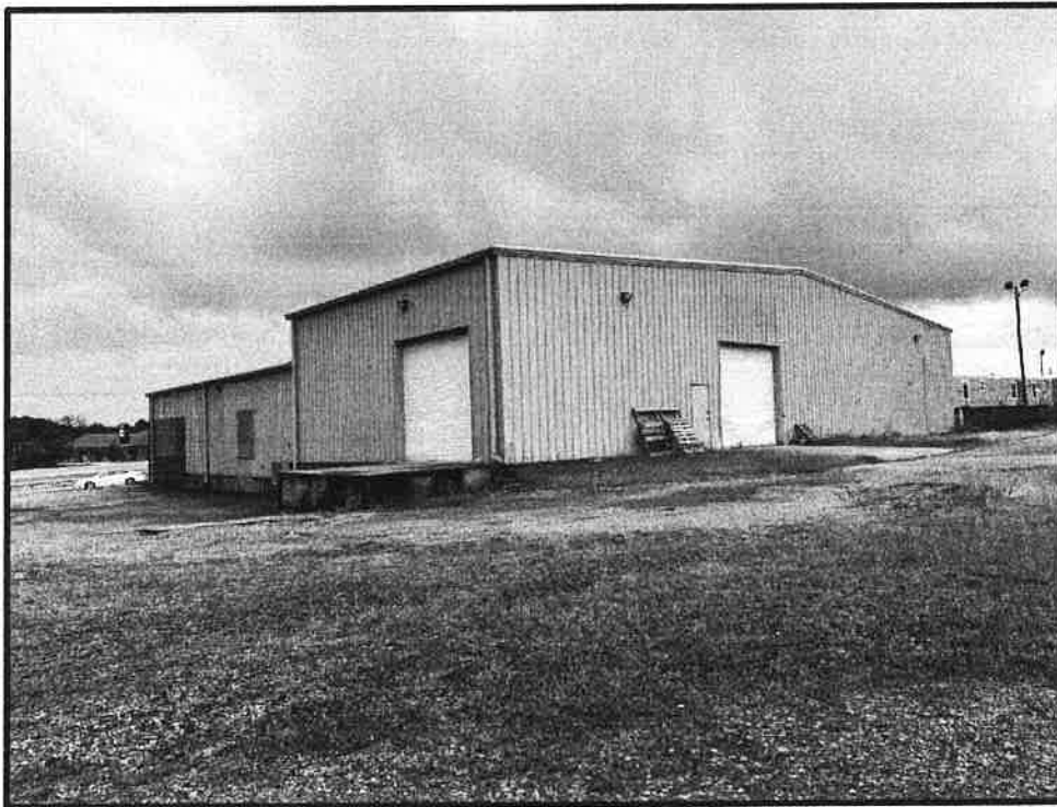
Rear view and northern elevations
