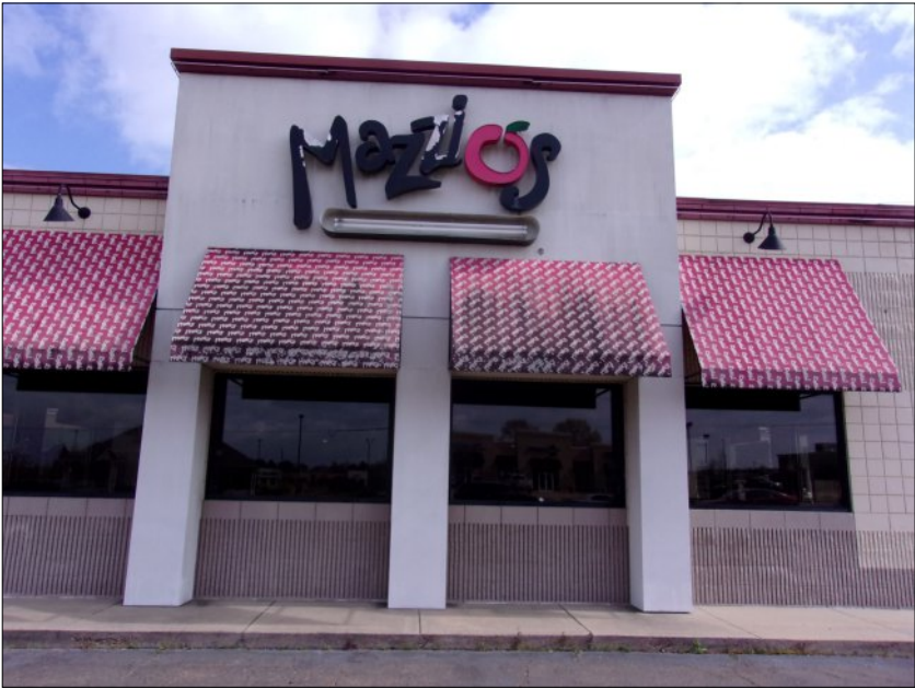
PHOTO SURVEY OF EXISTING - NORTH
