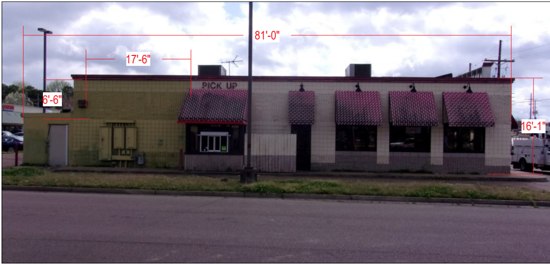
PHOTO SURVEY OF EXISTING - EAST Scale: 1/16" = 1'-0"
